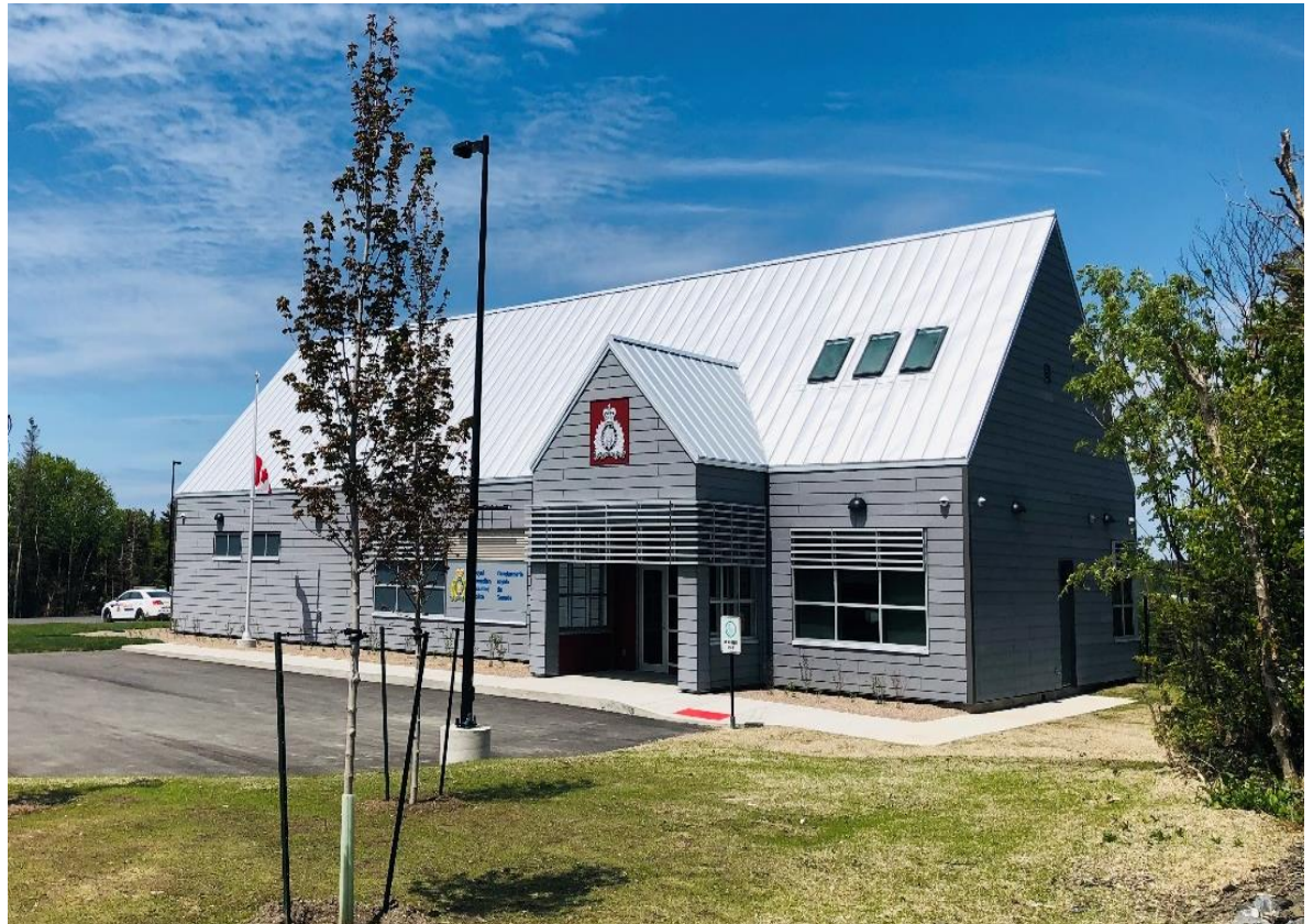
Opened in 2021, RCMP's Rocky Harbour (NL) Detachment is a Net-Zero Carbon Ready building that include state-of-the-art thermal design, automated lighting and plumbing fixtures (Photo Credit: A Simpson).
