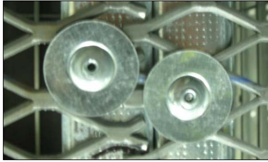
Figure 5: Example of Mesh Interlay Seam, Riveted
